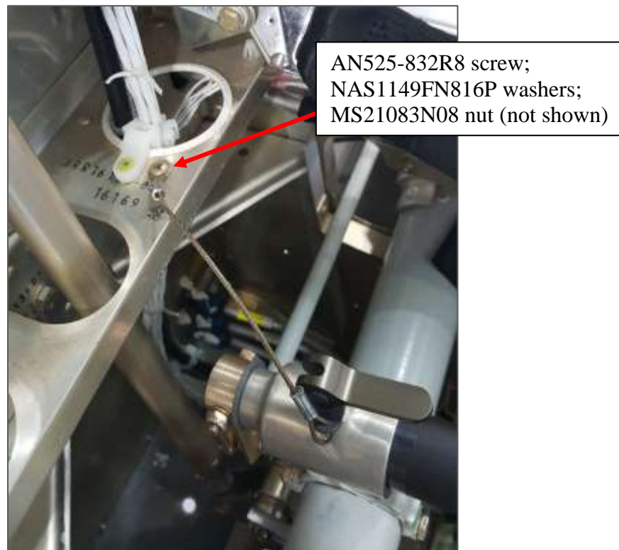
Figure 1. Former Retention Pin Lanyard Installation
