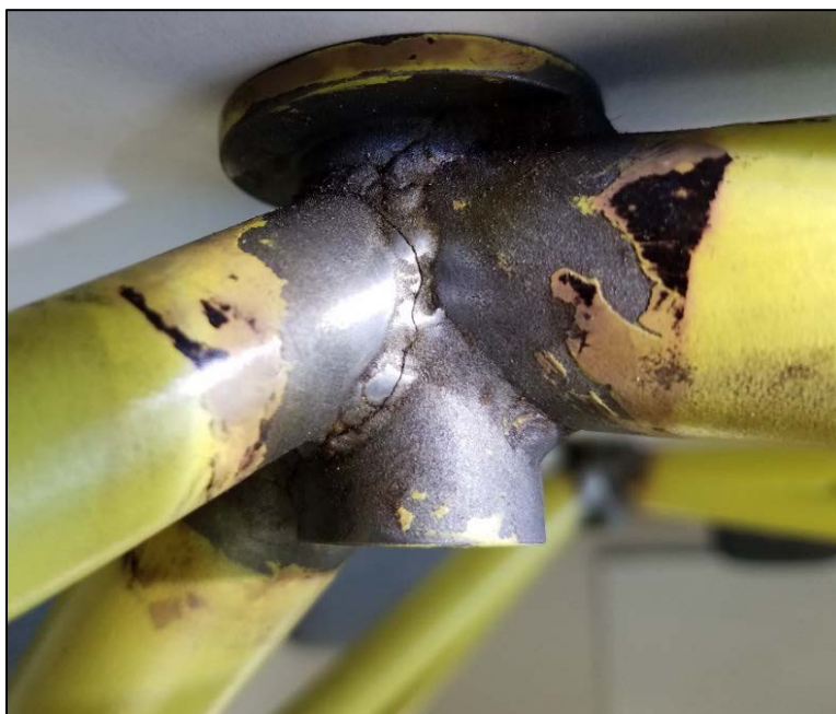
Figure 4. Photograph of Cracked Area – Forward Left Mount (Same area as in Figure 2 except mirror was not used; paint/epoxy primer removed)
