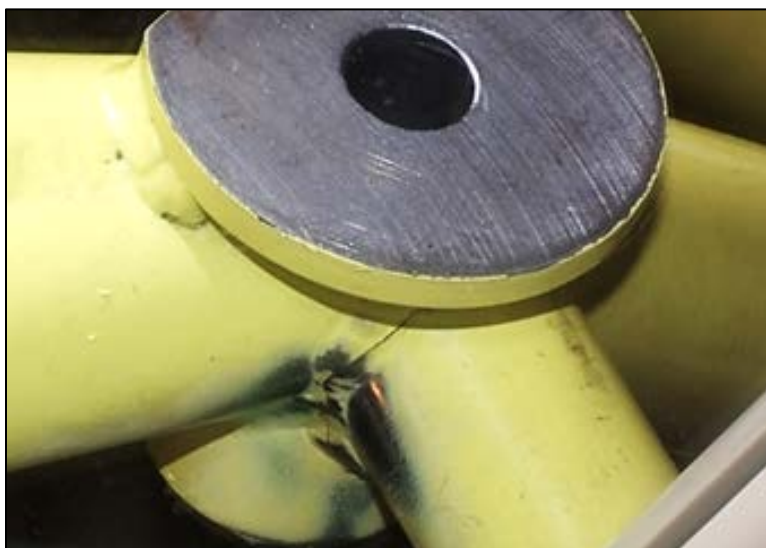
Figure 2. Photograph of Cracked Area – Forward Left Mount (Photo taken using a mirror)
